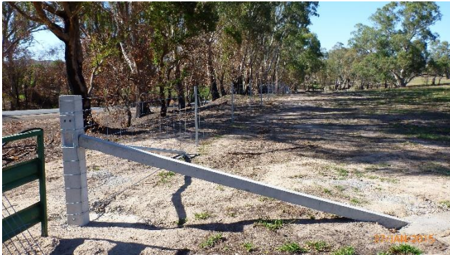
PHOTO: Concrete strainer post on a boundary fence.
