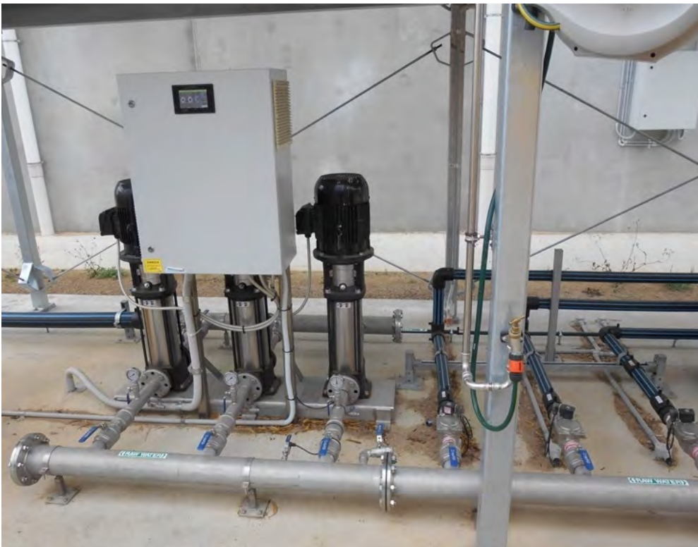
Photo 12: Murray Bridge truck wash pressure pump and supply manifold, including backup pump
