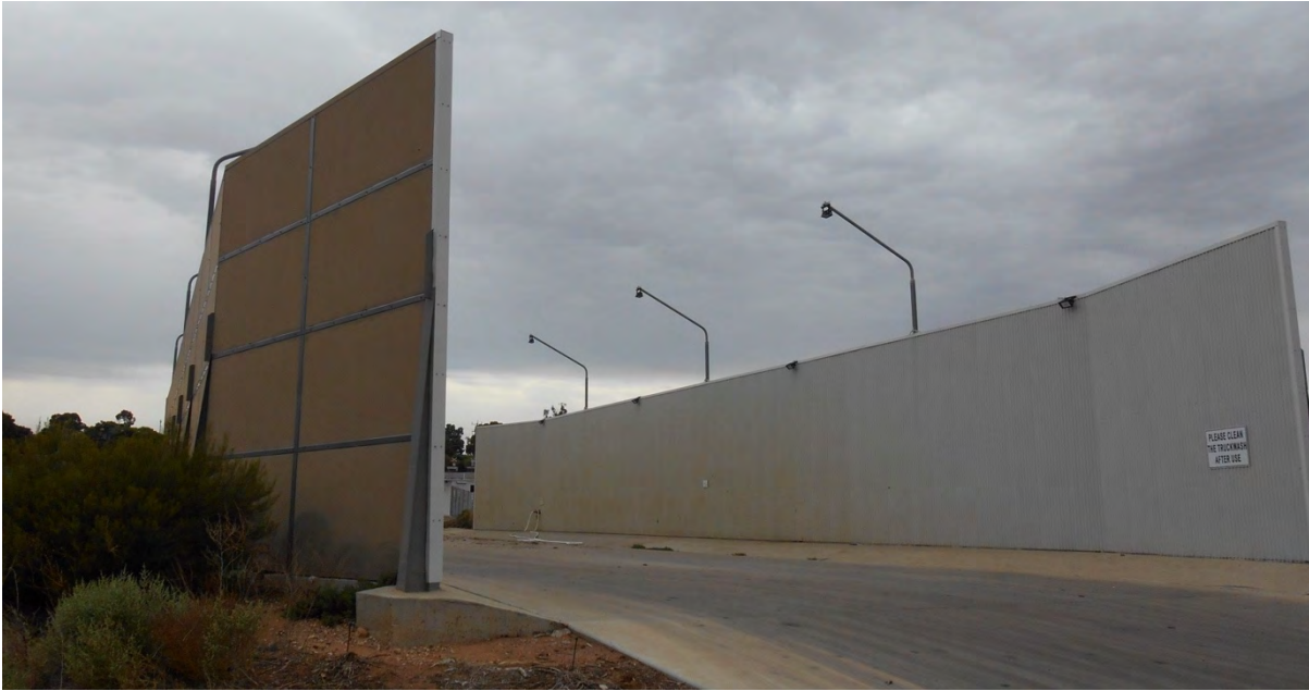
Photo 5: Ouyen truck wash showing walls, lighting, slope and water hose
