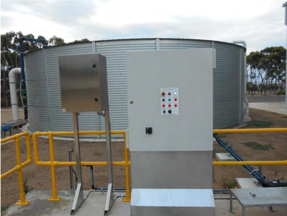
Photo 13: Supply tank (250,000 L) providing primary treated Murray River water for the truck wash
