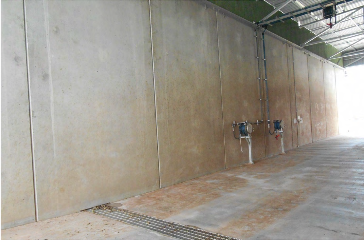
Photo 9: Murray Bridge truck wash showing concrete floor with grated main drain, concrete walls, steel roof, main wash reels (wall and roof mounted) and wall-mounted disinfectant reel
