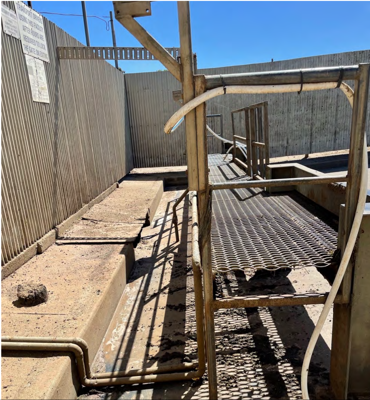
Photo 20: Geelong truck wash drains and piping
