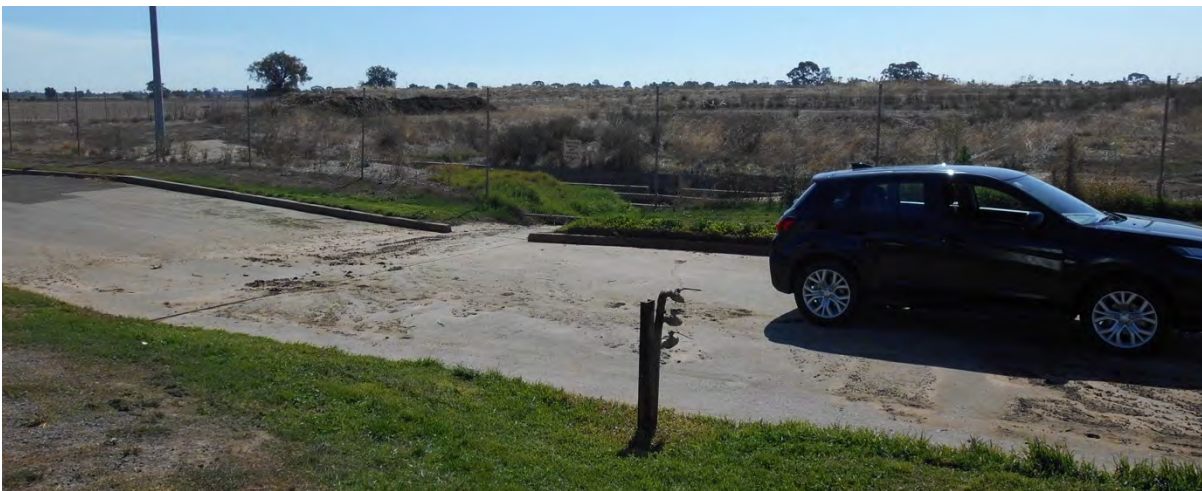
Photo 1: Horsham truck wash bay and effluent pits indicating narrow bays and no separation between two bays
