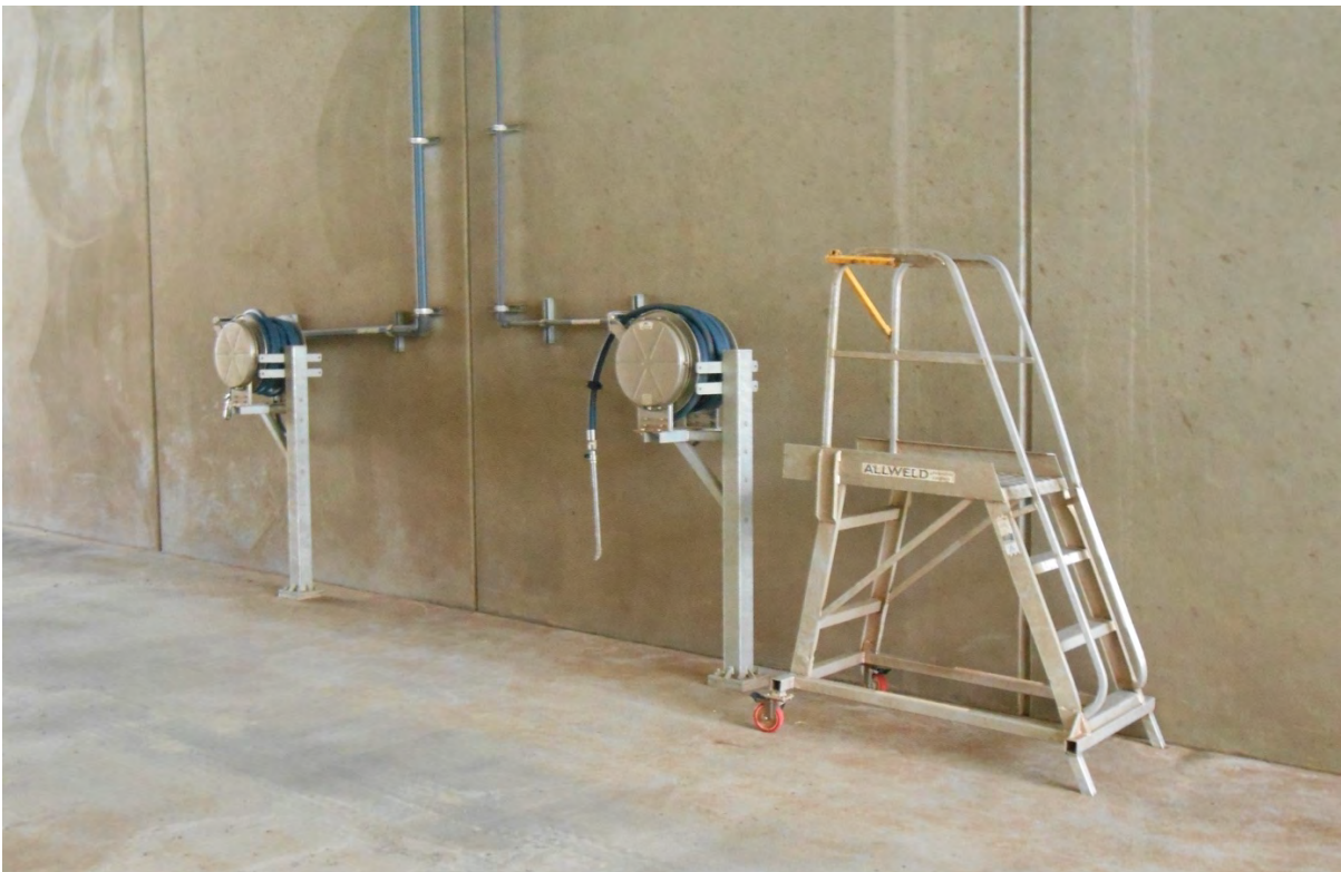
Photo 10: Murray Bridge truck wash showing wash reels and safety step ladder and platform
