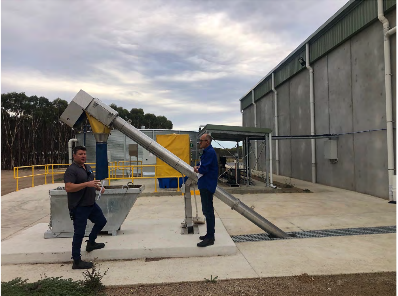
Photo 11: Murray Bridge truck wash showing solids removal auger and modular skip for removal off-site
