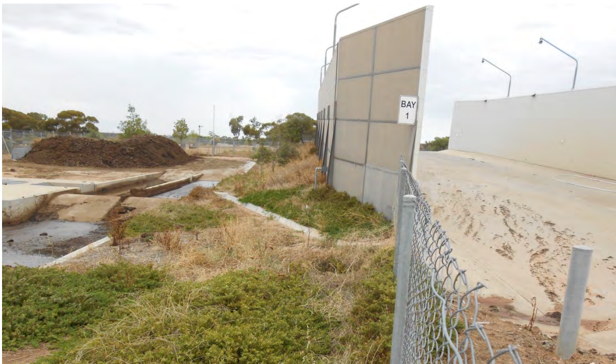
Photo 4: Uyen truck wash bays, effluent channel and effluent pre-treatment area
