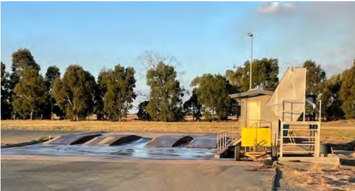
Photo 16: Echuca Truck wash showing poor slab slope and retrofitted raised bays
