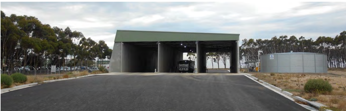
Photo 7: Murray Bridge truck wash showing bays, stormwater pit and water storage tank
