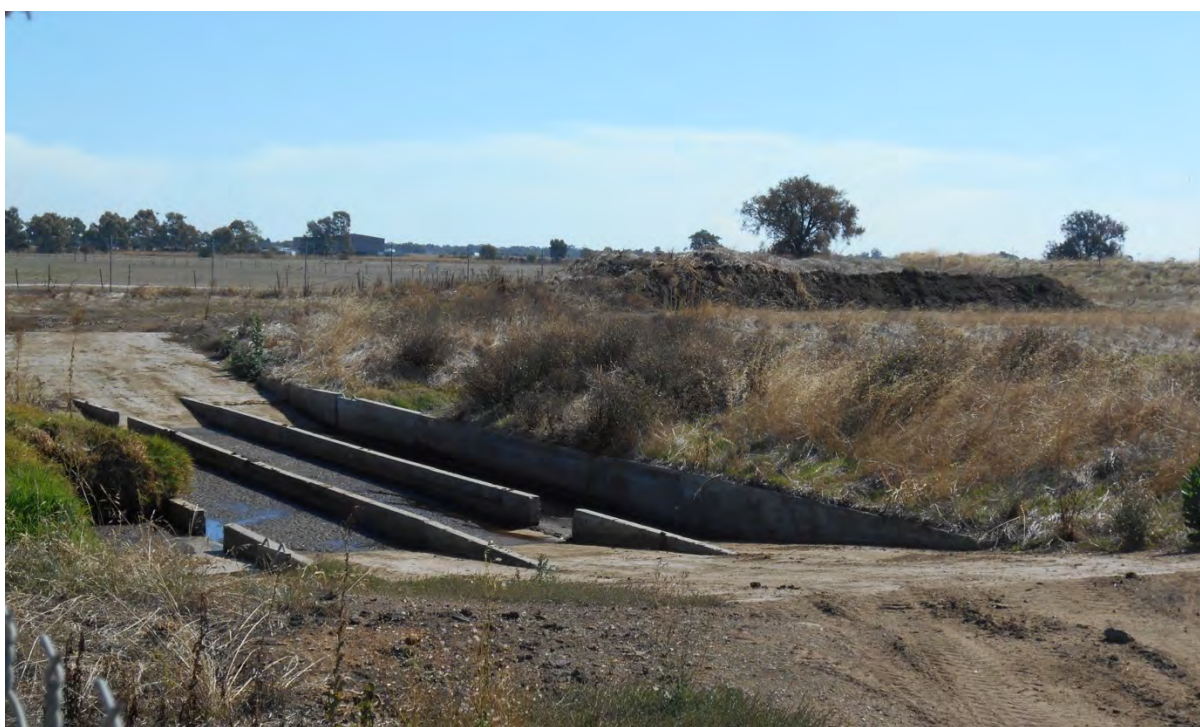
Photo 3: Baffled setting area within wastewater management system to enable ease of removal of dried solids stockpiled in the background
