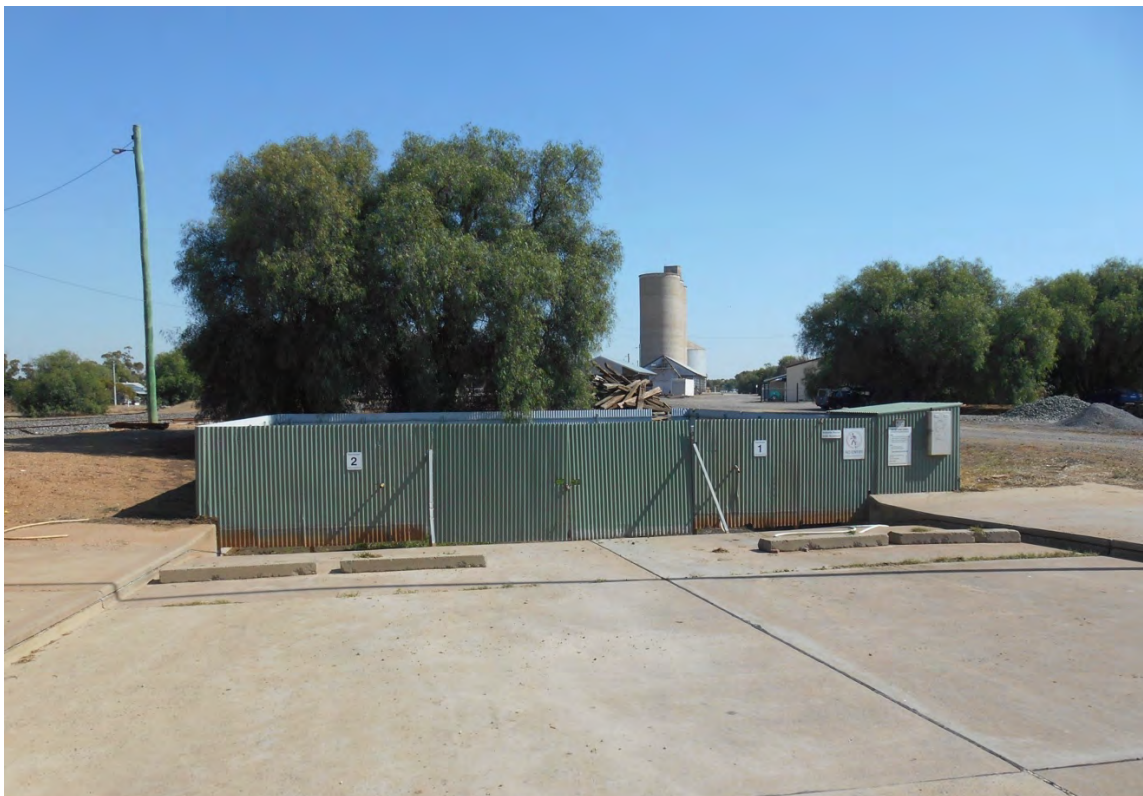
Photo 15: Wycheproof truck wash showing concrete washdown aprons in foreground, lights and fenced wastewater collection area
