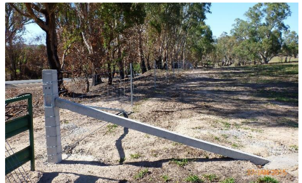
Concrete strainer post on a boundary fence
